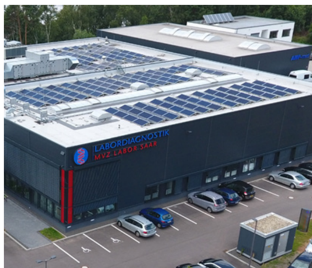
Solar panels on Labdiagnostik’s purpose-built laboratory in St Ingbert, Germany
